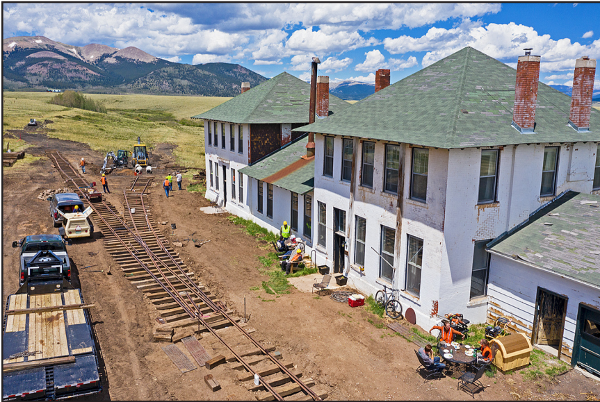
Denver, South Park & Pacific Historical Society volunteers built additional narrow gauge track on the Denver, South Park & Pacific Railroad right of way June 27, 2020, north of the Como Hotel in Como, Colorado. This track was originally abandoned in 1938 during the Great Depression.– Photo © 2020 by Chip.
