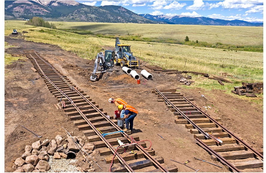
Narrow gauge track construction on June 27, 2020 included a new culvert at lower left. The right of way at left led to Boreas Pass and Breckenridge, Colorado, (Track No. 39 on map below). The track to the right led to Kenosha Pass and Denver. The grade is visible at upper center going right. – Photo © 2020 by Chip.
